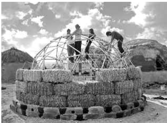
Straw-bale, earth-plastered domes being built on geodesic frames will become student housing at Kibbutz Lotan's Center for Creative Ecology, Israel.
